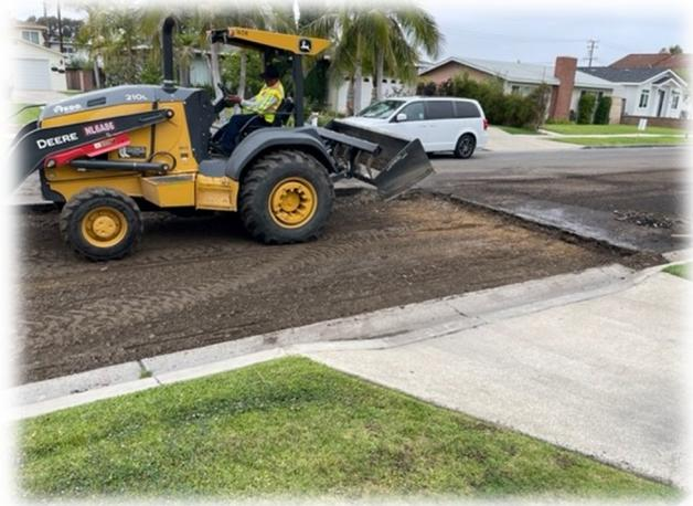
Photos: (Clockwise: left to right) Street grinding and overlay of a residential street
